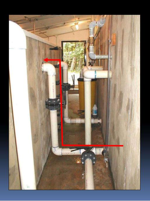
Telescoping valve with a V-notch weir serves the same function as an effluent weir.
