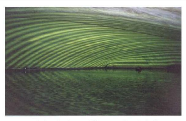
Plate 2.2 - Internal view of a slow sand filter covered by plastic film supported by positive air-pressure at Walton, Thames Water
