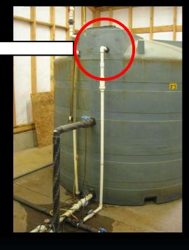
Some systems use influent float control valves in order to control the headwater level above the sand. This shows the location of the inlet float control valve on the inside of a small package filter.
