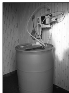
Diaphragm pump with chlorine solution tank
