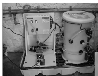
Erosion chlorinator
